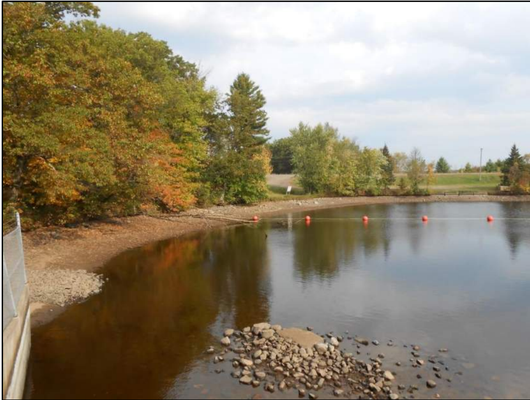
Figure 3.1.3-3 Take-Out Facing North from Spillway
