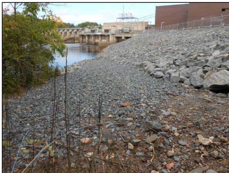
Figure 3.1.6-2 East Tailwater Shoreline Facing Northeast
