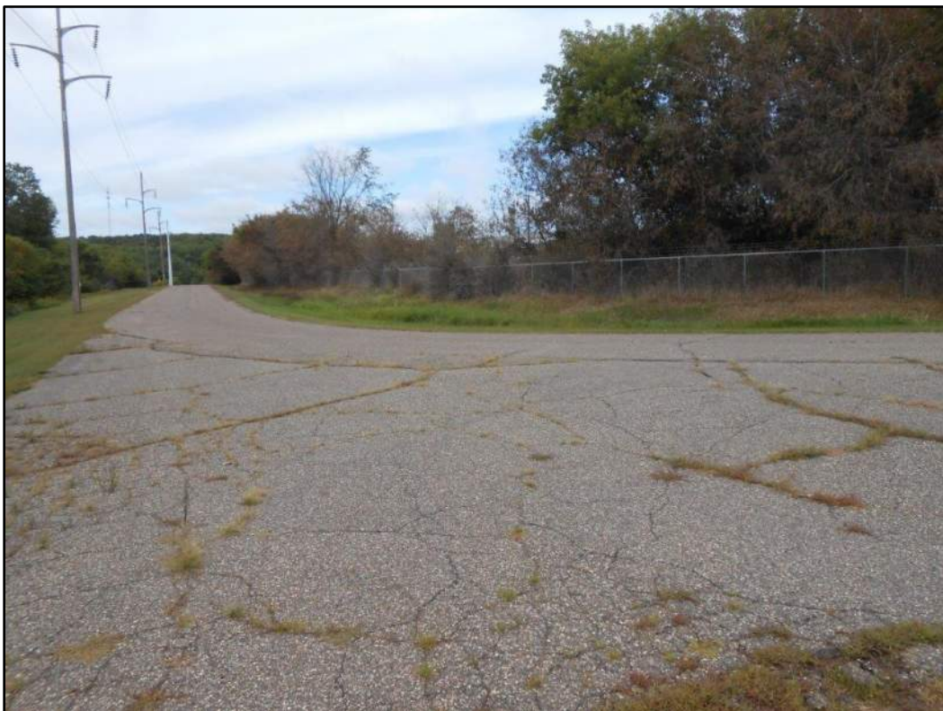
Figure 3.1.6-6 Access Road to East Tailwater Shoreline Facing West
