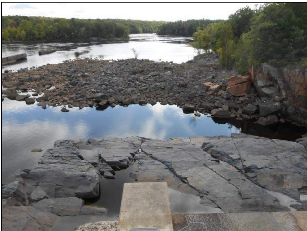
Figure 3.1.7-2 West Tailrace Fishing Access Photo Looking South Below Dam
