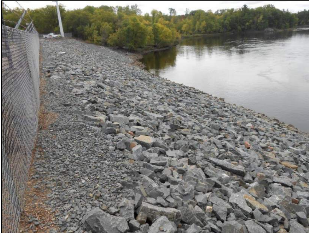
Figure 3.1.6-3 East Tailwater Shoreline Facing South
