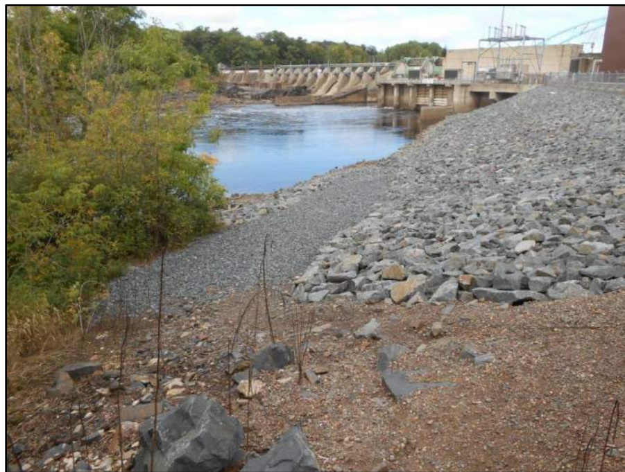
Figure 3.1.6-1 East Tailwater Shoreline Facing North
